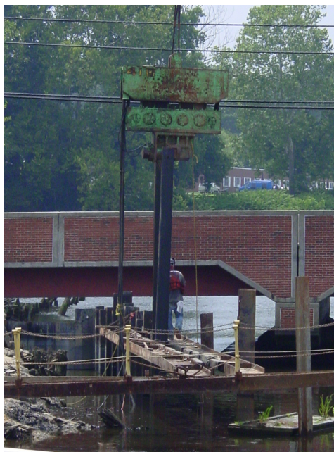
Steel sheet pile installation
