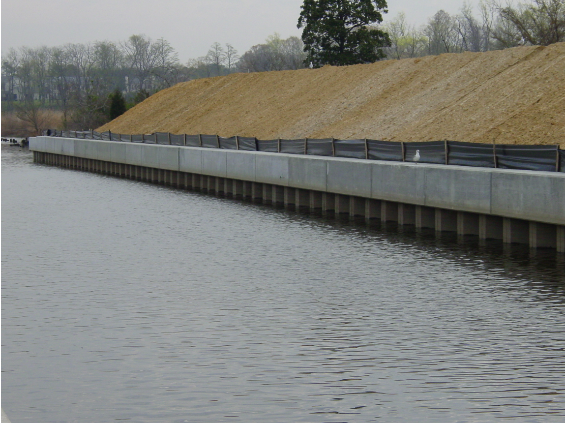
Steel sheet pile bulkhead with soil surcharge loading
