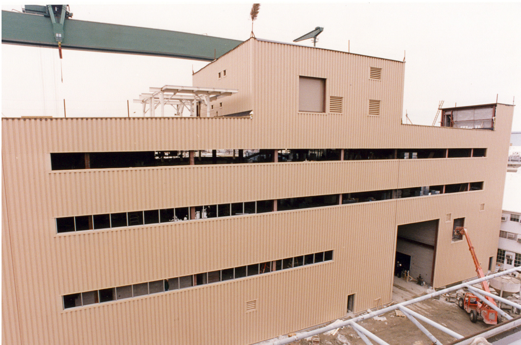
Exterior View – Installation of siding
