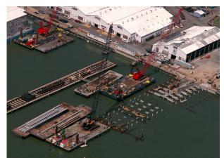
Concrete pile installation and precast cap placement
