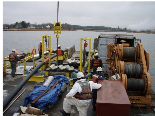
Crews installing concrete weights as the pipelines are deployed from the laybarge
