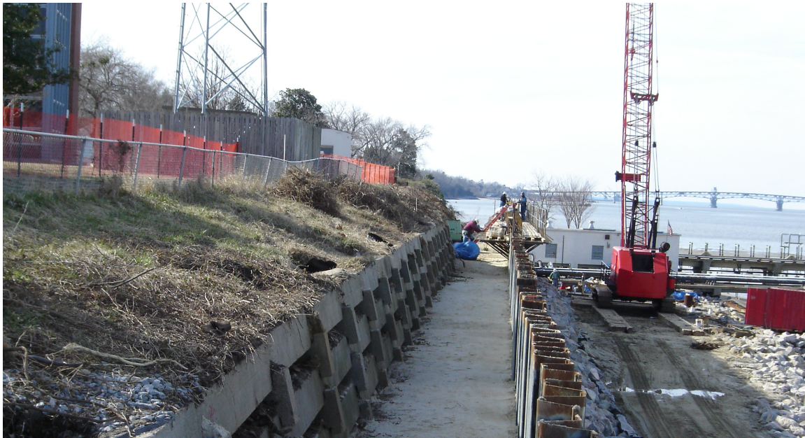
Construction of the concrete cap for the steel sheet pile bulkhead
