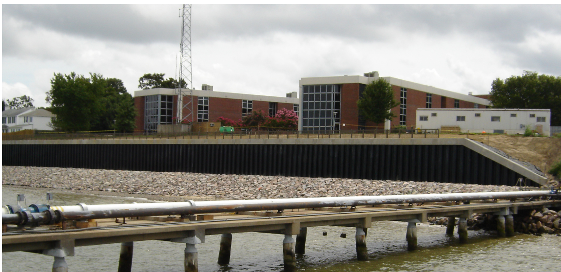
Steel sheet pile bulkhead with concrete cap, soil cement anchors, and customized handrail
