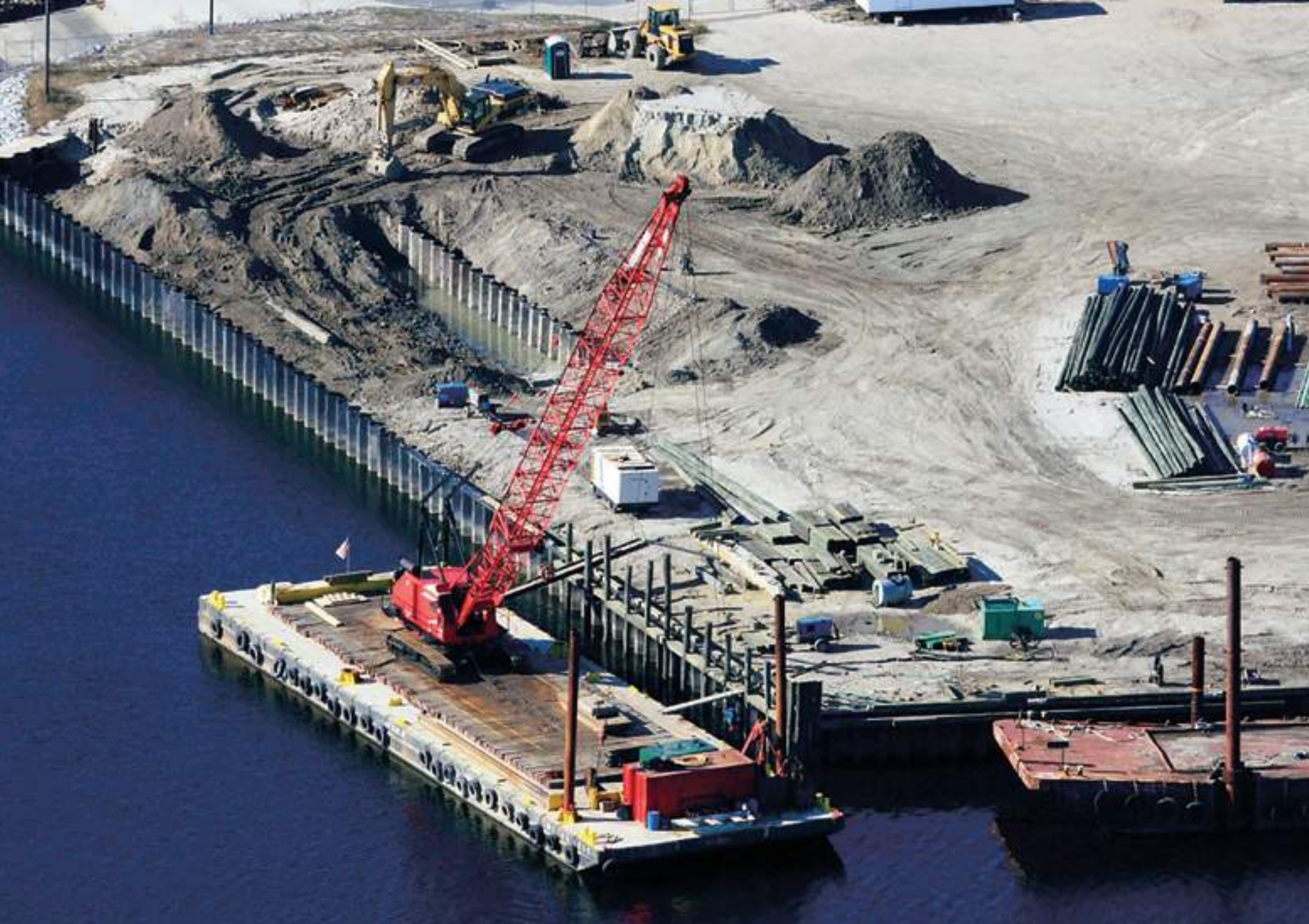
Norfolk dredge bulkhead
