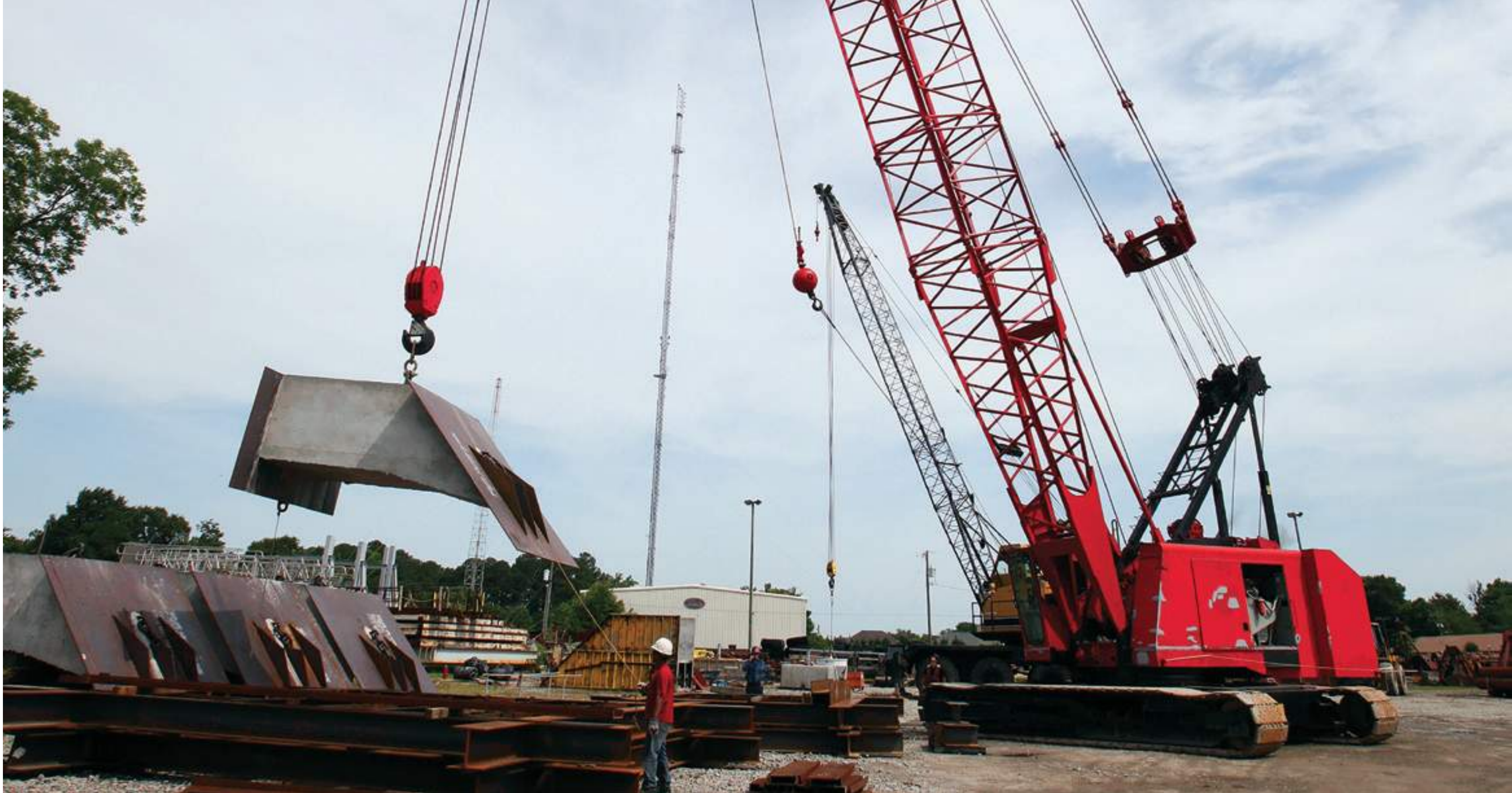
Casting 72,000-pound anchors for security barriers.
