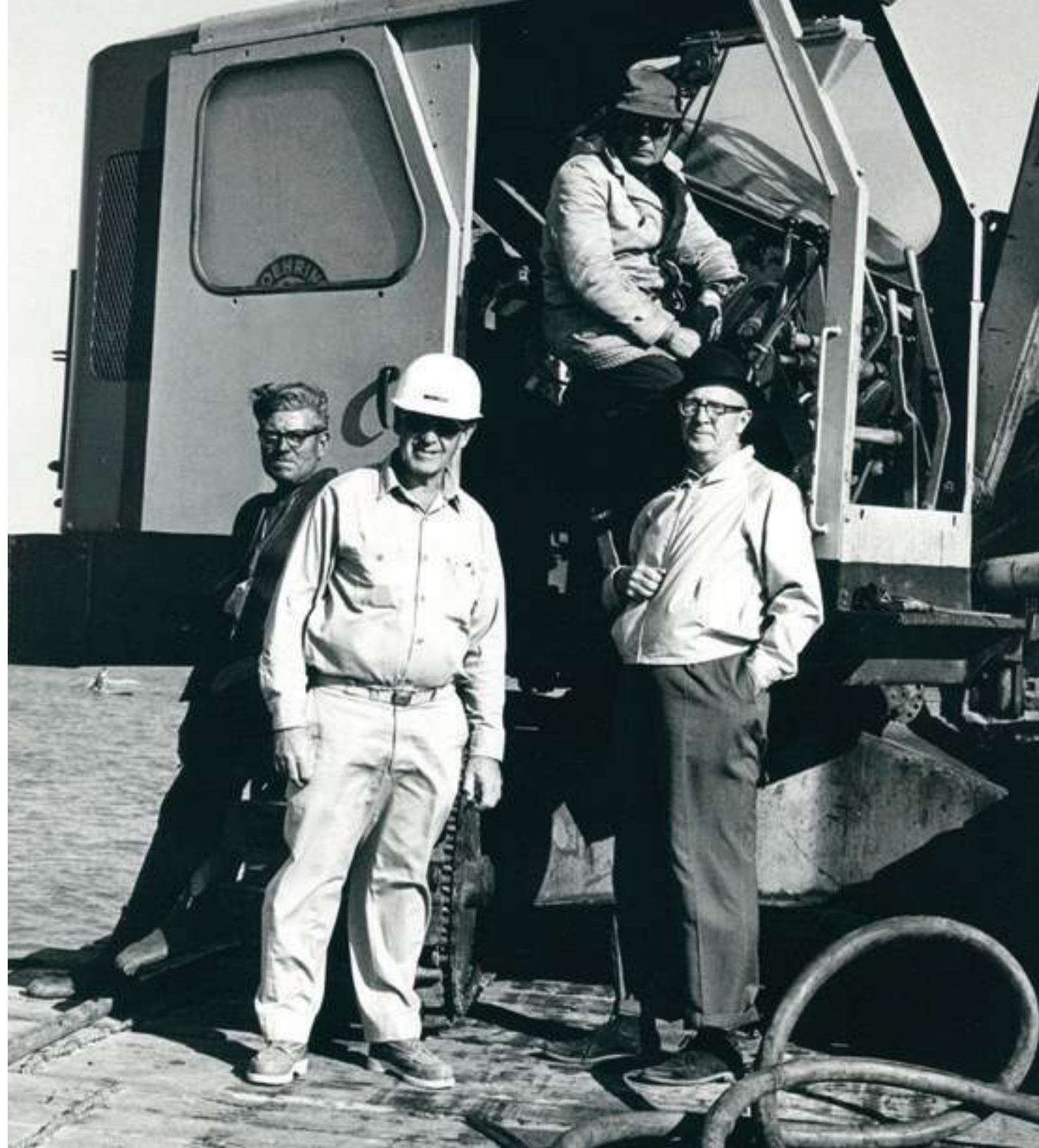
Rudee Inlet Rip Rap Protection (1967)
