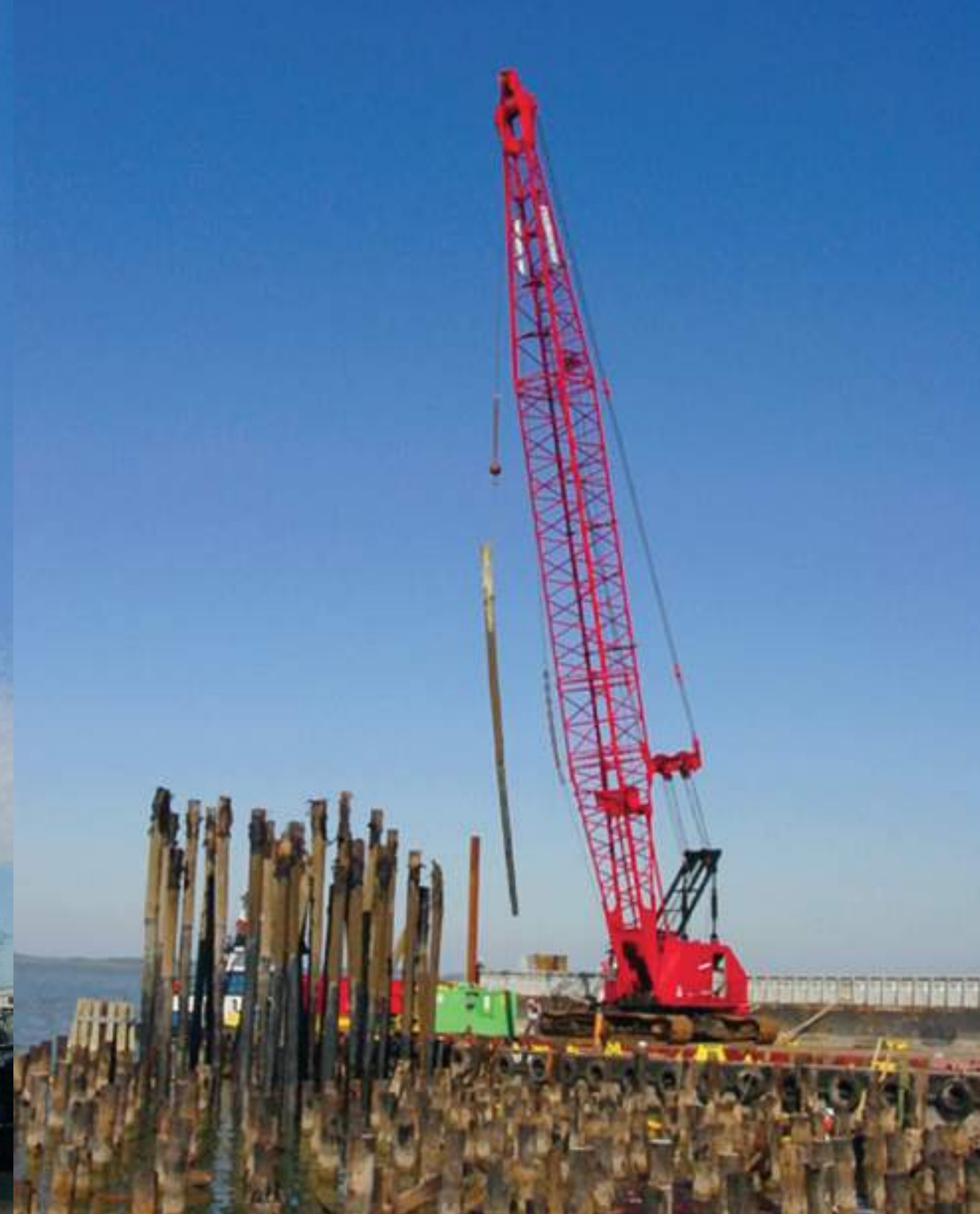
Pier demolition at Fort Eustis, VA
