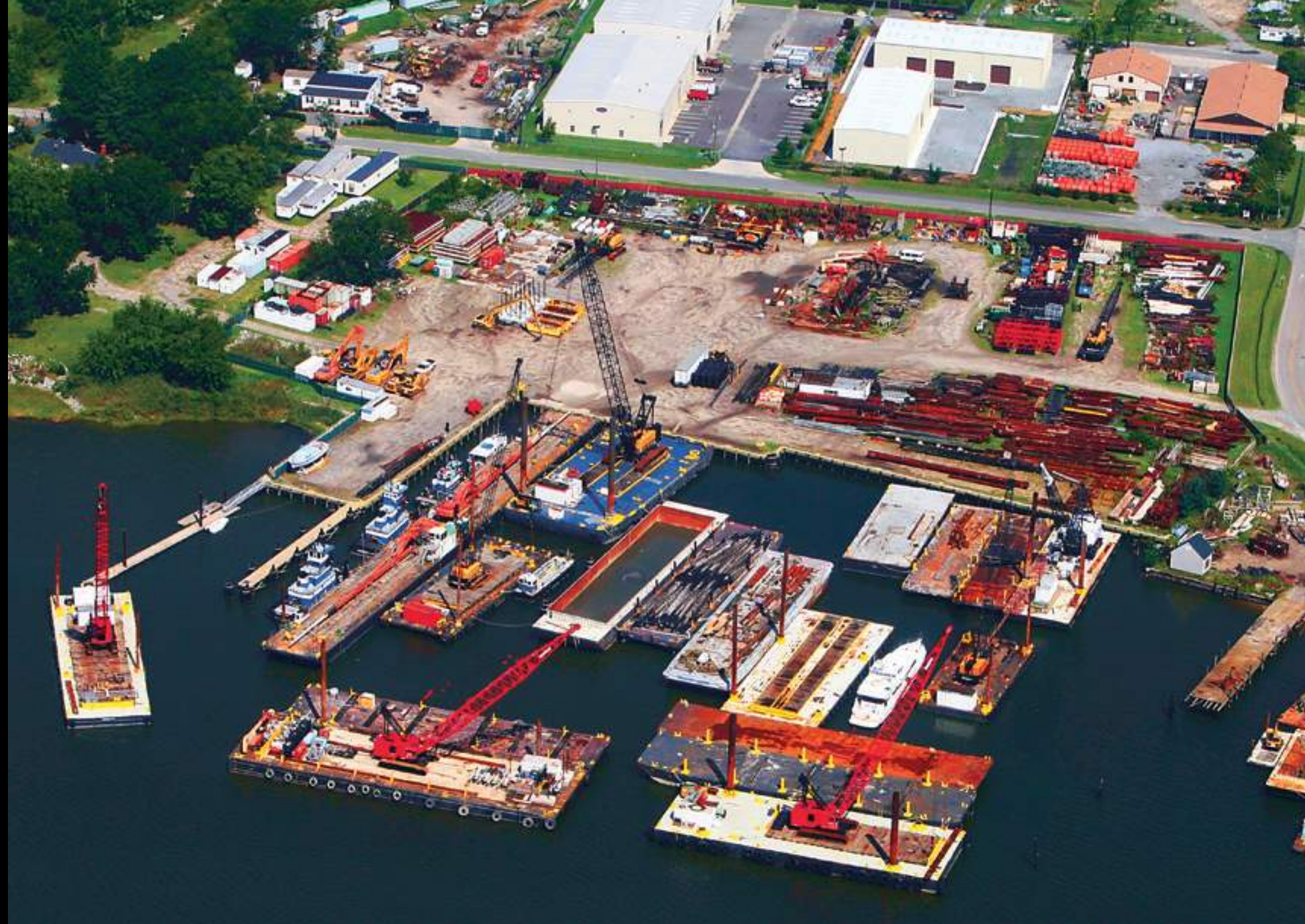
WFM Construction Yard, Portsmouth, VA
