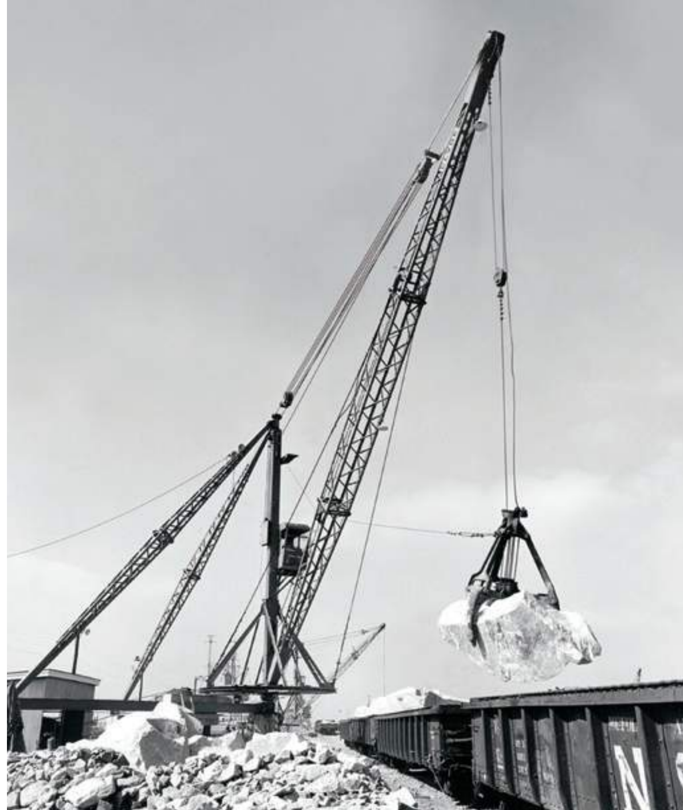
Chesapeake Bay Bridge Tunnel Unload Rip Rap for Southern Materials (1960s)
