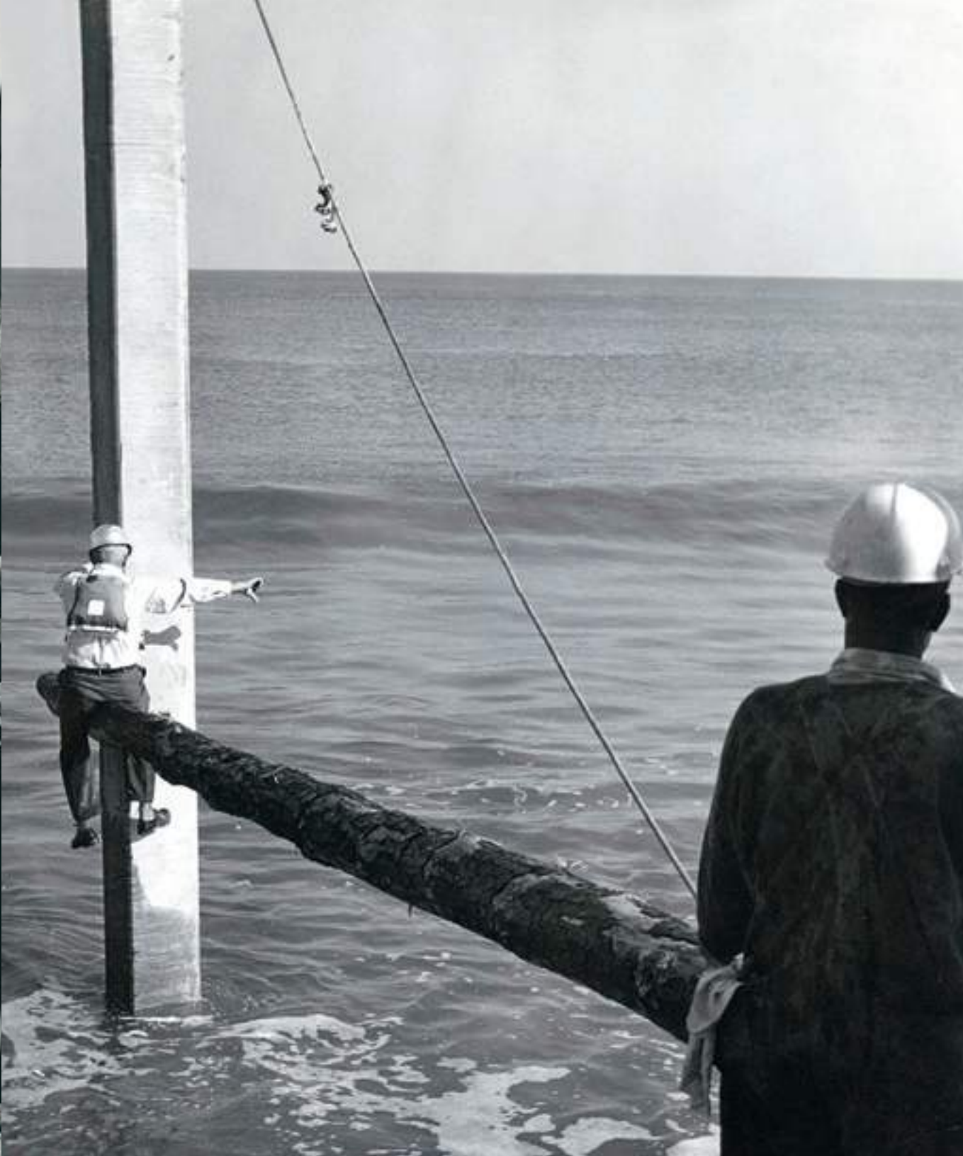
Rudee Inlet Rip Rap Protection (1967)
